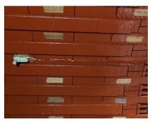
IRIS POWER FFPROBE INSTALLED ON A TURBINE GENERATOR STATOR WEDGE
