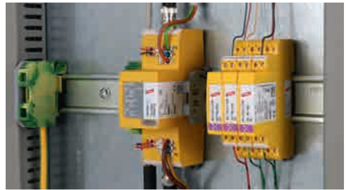
Space-saving and application-optimised 3in1 DEHNvario arrester for analogue camera systems.
