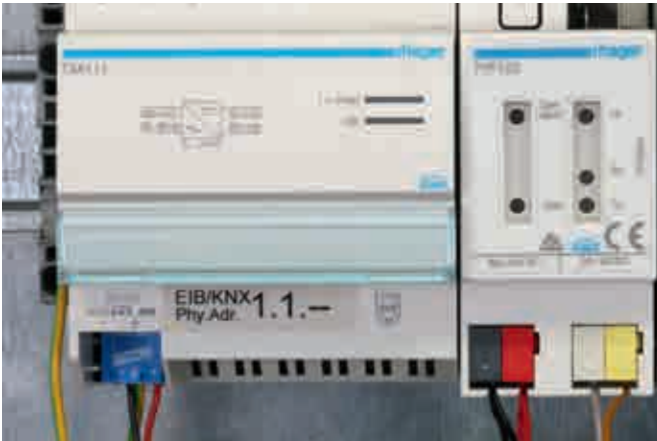
Protection of a KNX power supply unit by means of a BUSector surge arrester mounted in the bus terminal slot.
