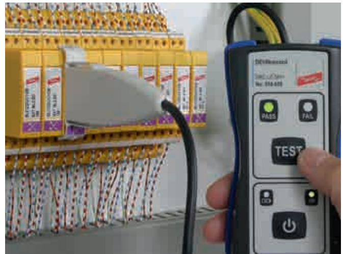
Testing a protection module via a hand-held device based on RFID technology (LifeCheck).
