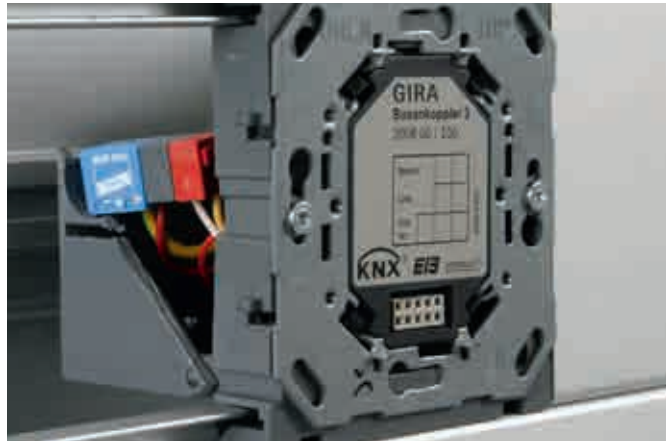
Protection of a KNX bus coupling unit by means of a BUSector surge arrester mounted on a bus terminal in the mounting panel of a cable duct.
