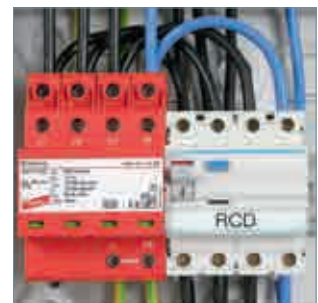
Series connection by means of a lightning-current-tested STAK 25 pin-shaped terminal
