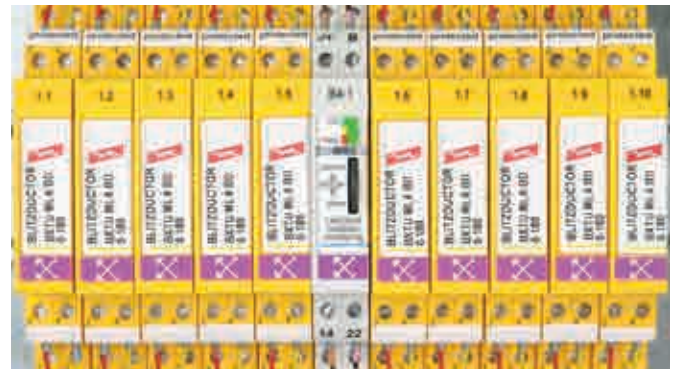
Installed DEHNrecord condition monitoring system
