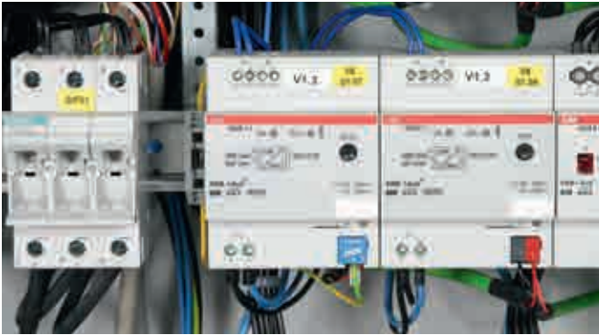
Surge arrester for KNX / EIB buses with connection wires.
