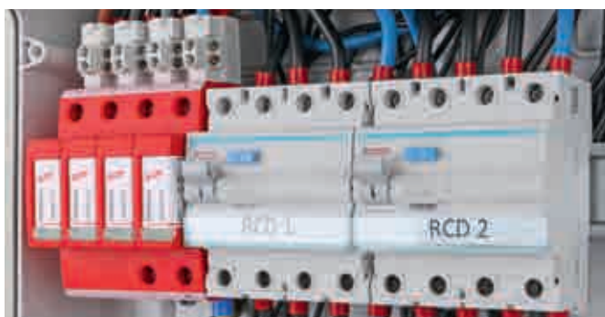
STAK 3X16 for EMC-optimised series connection of string lines in a PV generator junction box.
