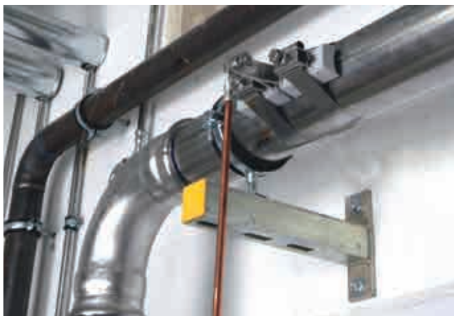
Installed at a StSt pipe.
