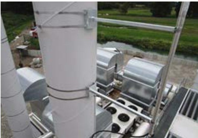
Spacer with tensioning strap fastener
